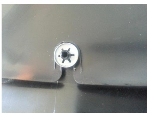
These two can be a little tricky to get off and easy to damage the old plastic bolts, but easier to get on to the new bolts.
